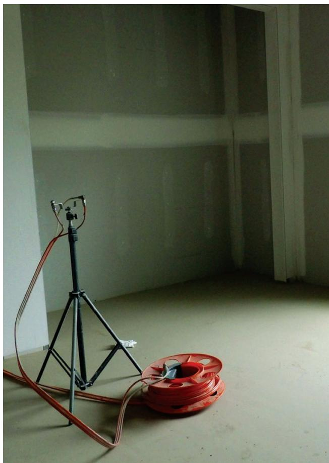
While a blower door pressurizes the house, emitter nozzles pump a fog of acrylic sealant into the building air. Walls can be exposed sheathing (above left) or finished with drywall (above right); either way, the aerosolized sealant flows out through any air leaks and coagulates on small openings as it encounters a reduction in temperature and humidity.
